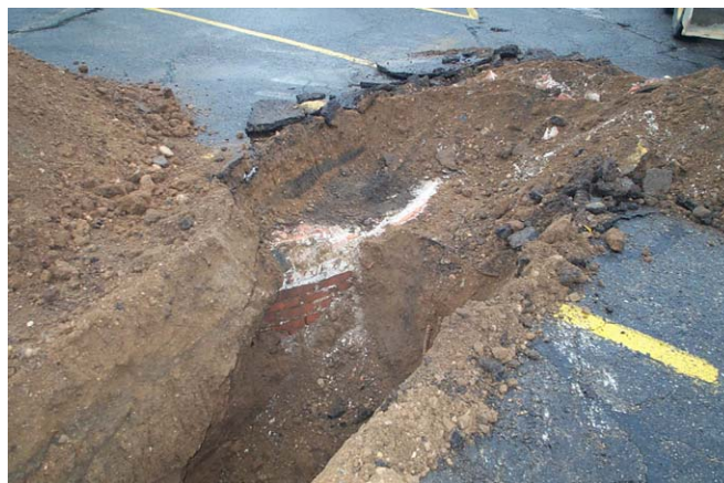
Figure 7. Excavation of former residential water supply cistern in Ann Arbor, Michigan.
