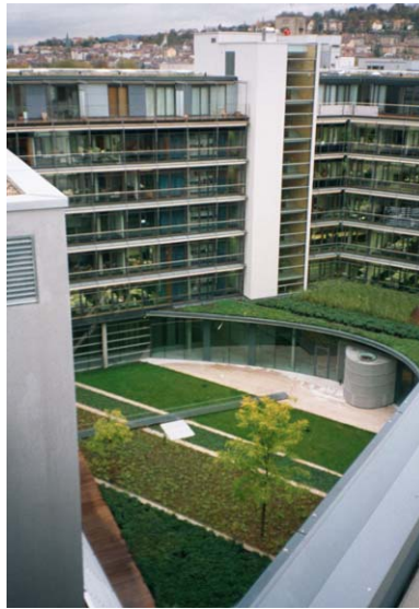
Figure 3. Vertical storage units for vegetated roof plaza maintenance are common in Germany
