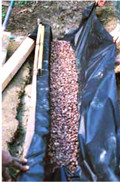
Figure 4. Construction of a French drain. ( www.gardenadvice.co.uk/howto/garden-build/frenchdrain/index.html )
