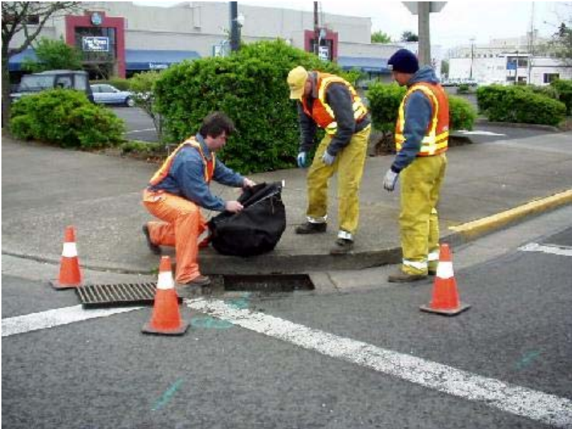
Figure 3. Filter Bag Installation (Full Circle Ag, Inc., http://www.fullcircleag.com/pages/954364/ )
