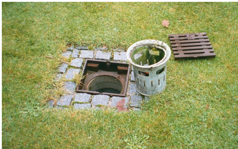
Figure 4. German basket-type water quality inlet example.
