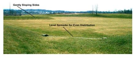
An Infiltration Basin is a shallow impoundment that stores and infiltrates runoff over a level, subtle, uncompacted, (preferably undisturbed area) with permeable soils.
